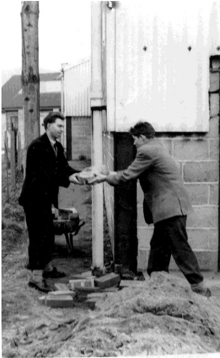
Above: David Warrington and Ken Pemberthy barrowing bricks c. 1957
